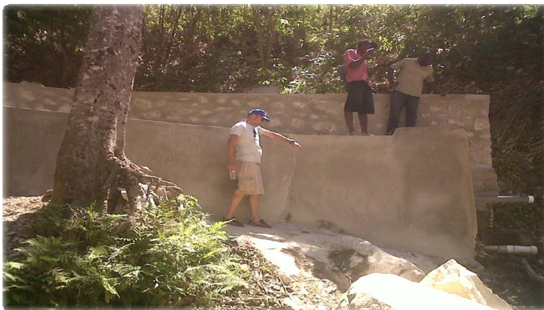
“Captage” system at a local spring, Cazale, Cabaret
